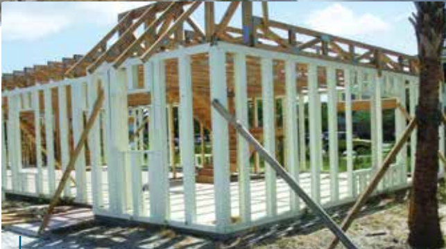
These condominiums in West Palm Beach, Fla., were constructed using wood floor and roof trusses and CBS’s first-generation pultruded composite profiles (in white) for the wall framing — assembled with metal screws rather than nails — on the first and second floors. Seven identical buildings were erected, illustrating how composite structural framing can be integrated with traditional wood-building methods. ■
